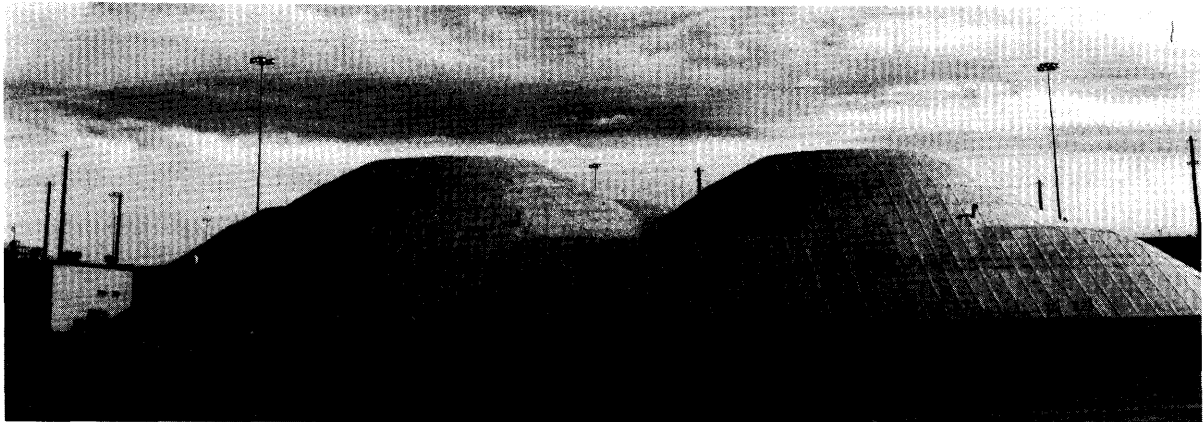
Explosion-resistant warhead disassembly cells at Pantex (Gravel Gerties).
